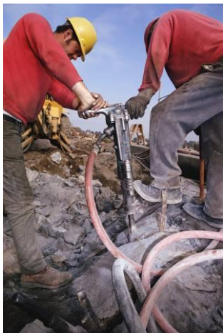
Example 1: Intense, repetitive and heavy physical workload
